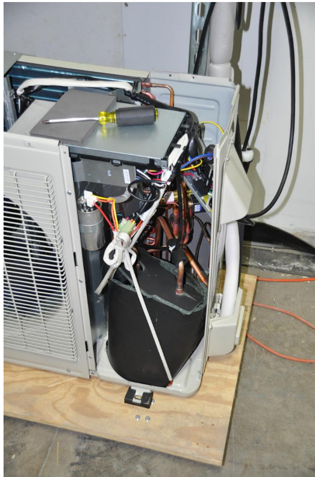
Picture of outdoor unit with side panel removed
